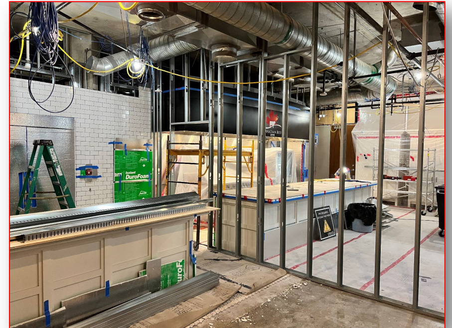
Multi-studio upgrades for CBCE takes shape
