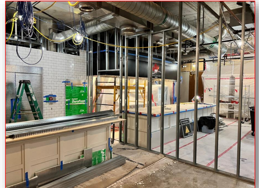
Multi-studio upgrades for CBCE takes shape
